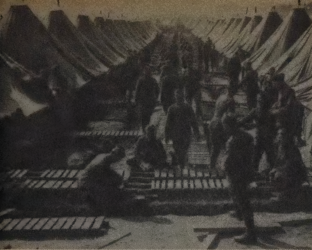
Mud at Camp Pontanezen [France] was made passable by laying sections of duckboards. Butler carried one in himself, earning the nickname "General Duckboard."
